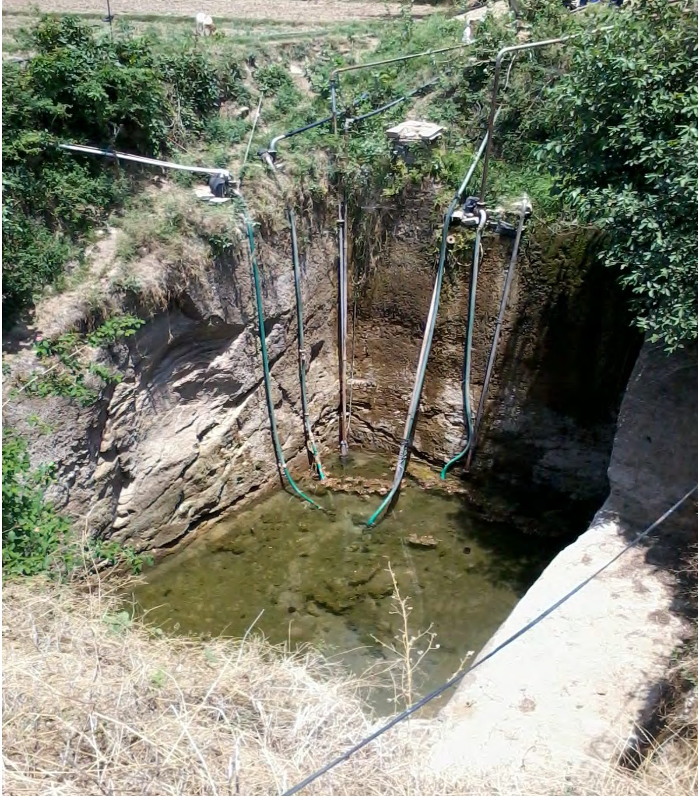
Shared open well with individual motors for pumping
